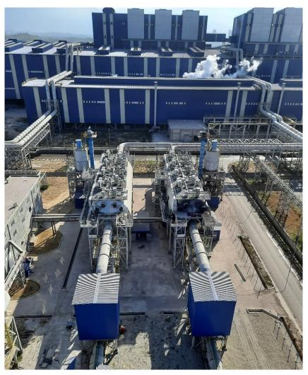
Environmental technology from SMS group: dry electrostatic precipitators of the latest generation.
