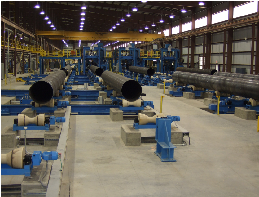
Picture, left: The space reserved for the fourth re-welding stand in Stupp Corporation's spiral pipe mill.
