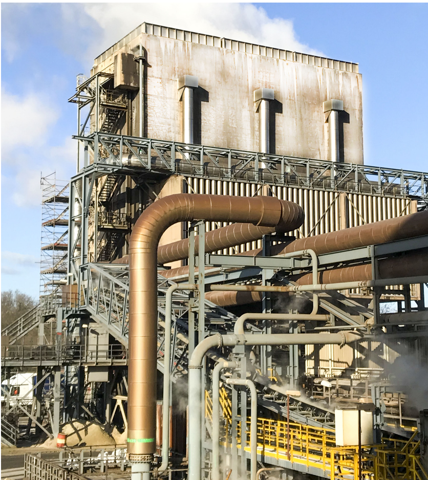
Modernised INBA ® plant at Rogesa's BF4.
